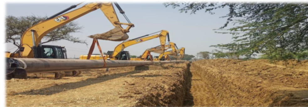
Setting up slurry pipeline
