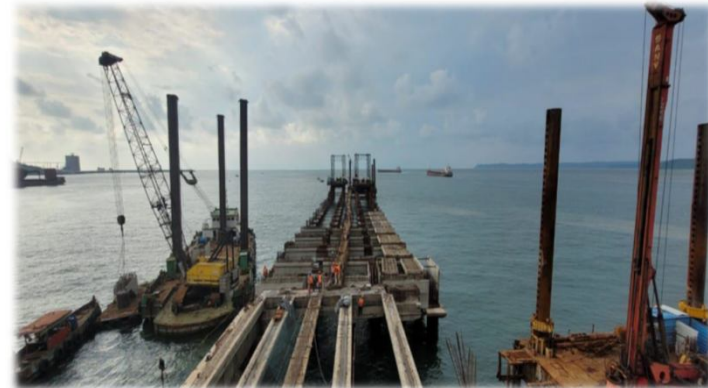
Approach Trestle & Berth in Progress
