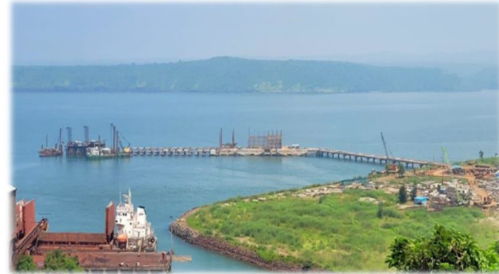
LPG construction at Jaigarh Port
