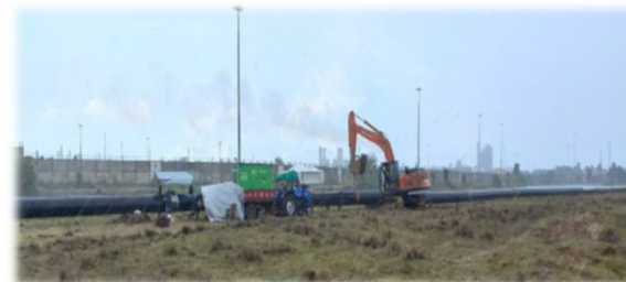
Setting up slurry pipeline
