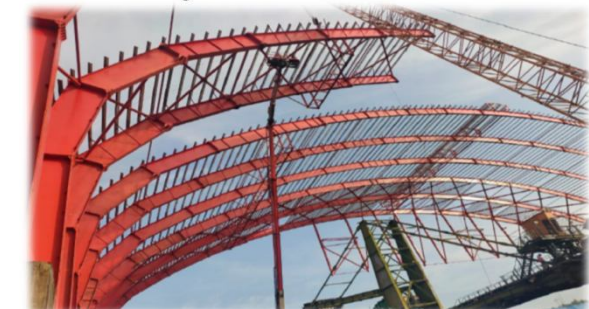
Work on Cover shed at South West Port, Goa
