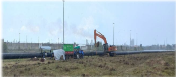
Setting up slurry pipeline
