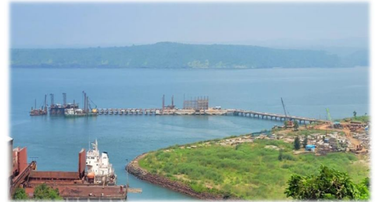
LPG construction at Jaigarh Port
